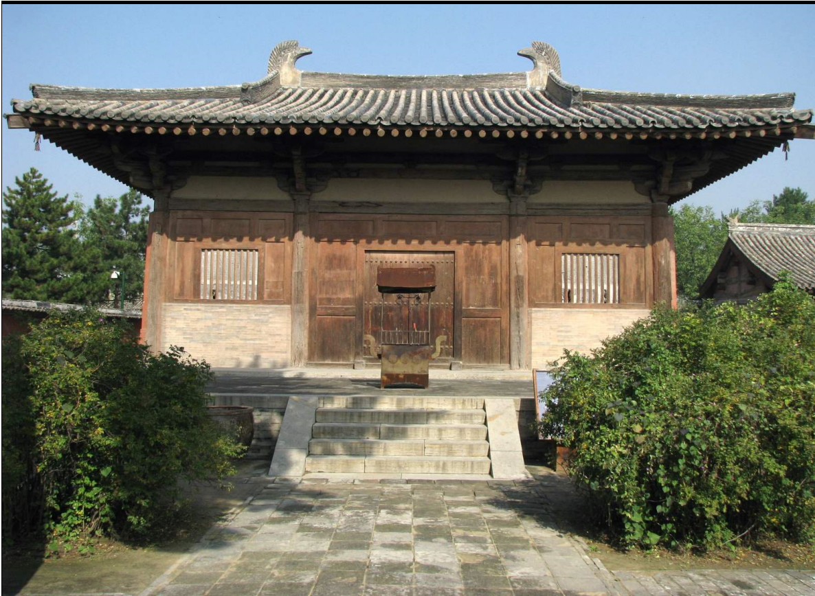
Main Hall, Nanchan Monastery Wutaishan, Shanxi Province, China, 782 CE
