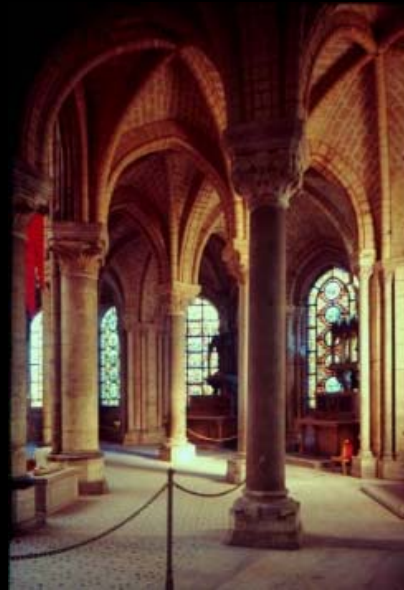
Substituted thin columns for heavy piers in the Ambulatory
