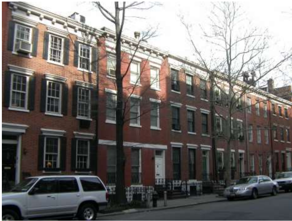
Charlton St houses, orig. built 1820s
