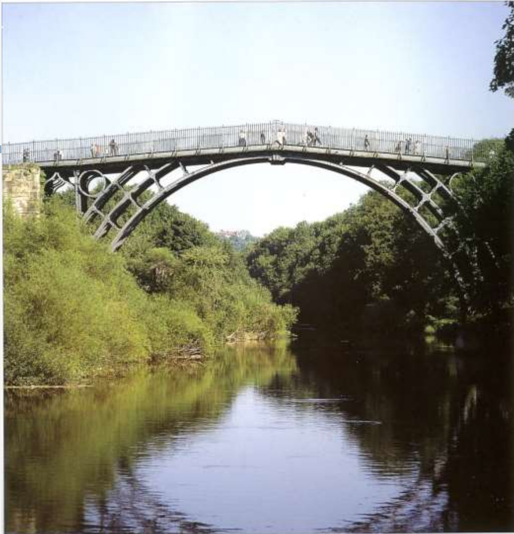
Coalbrookdale Iron Bridge Abraham Darby
