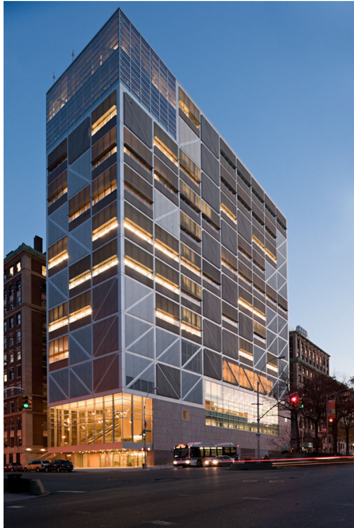
Northwest Corner Building, Columbia University, NY, NY 2008
