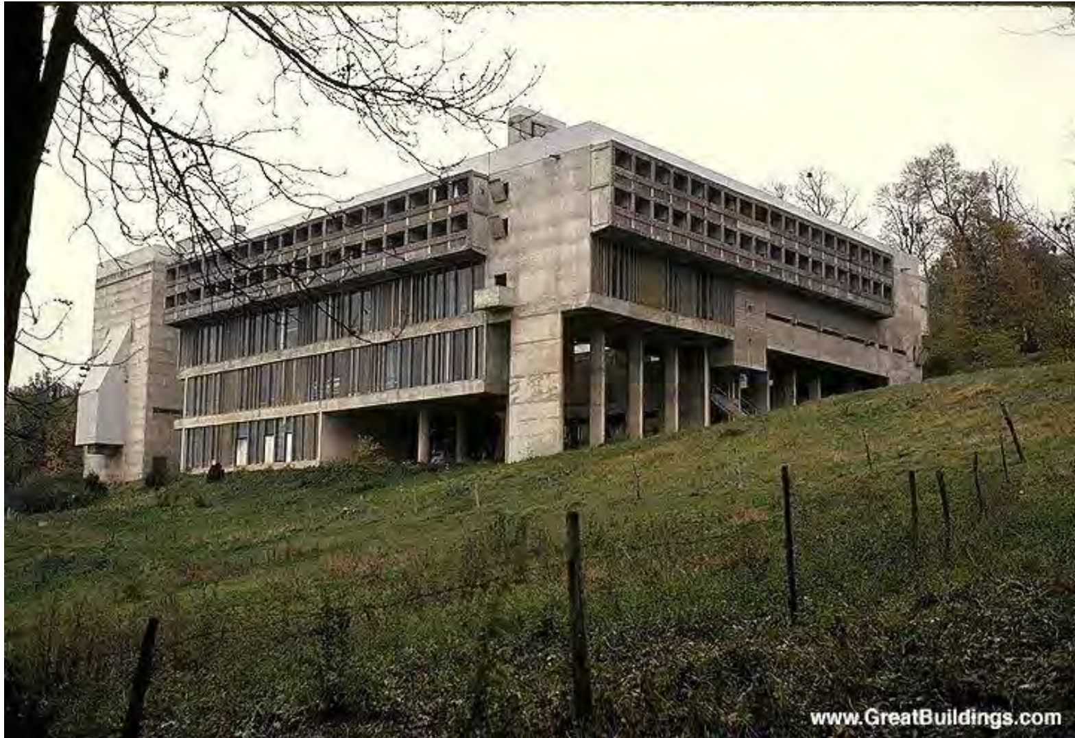
Monastery of La Tourette, (near Lyon) France 1953-60
