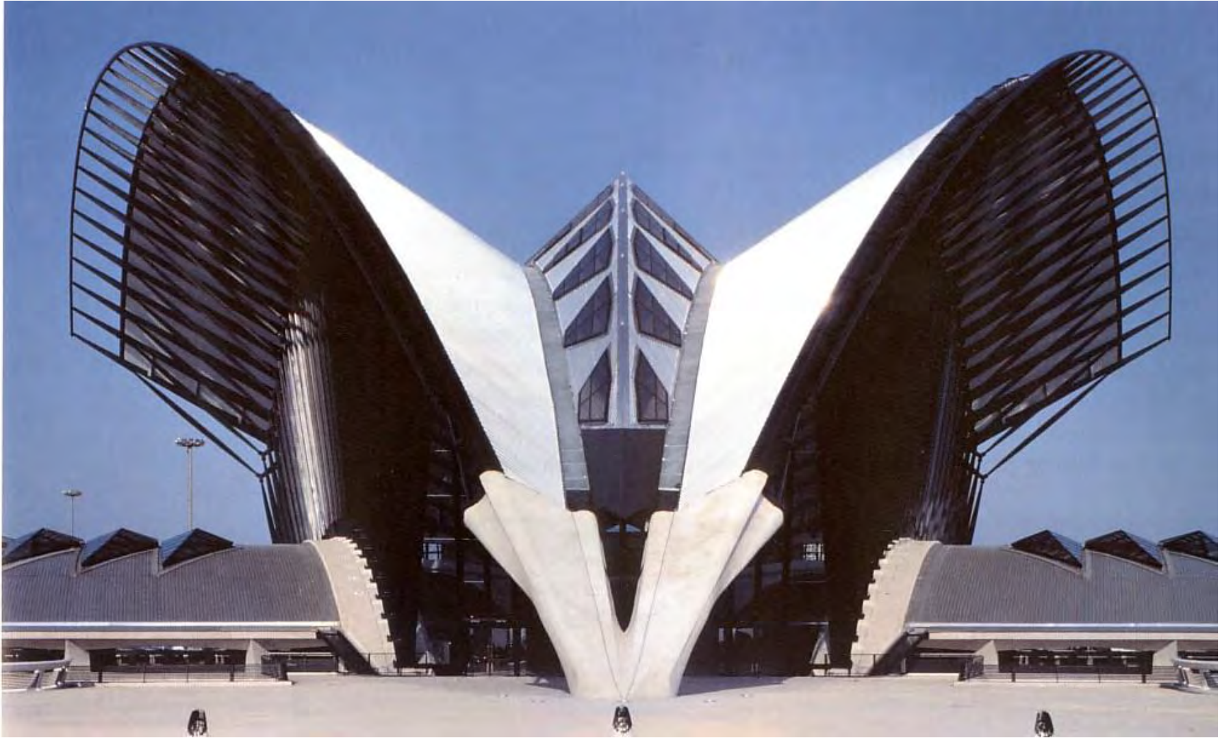
TGV Station, Lyon, France
