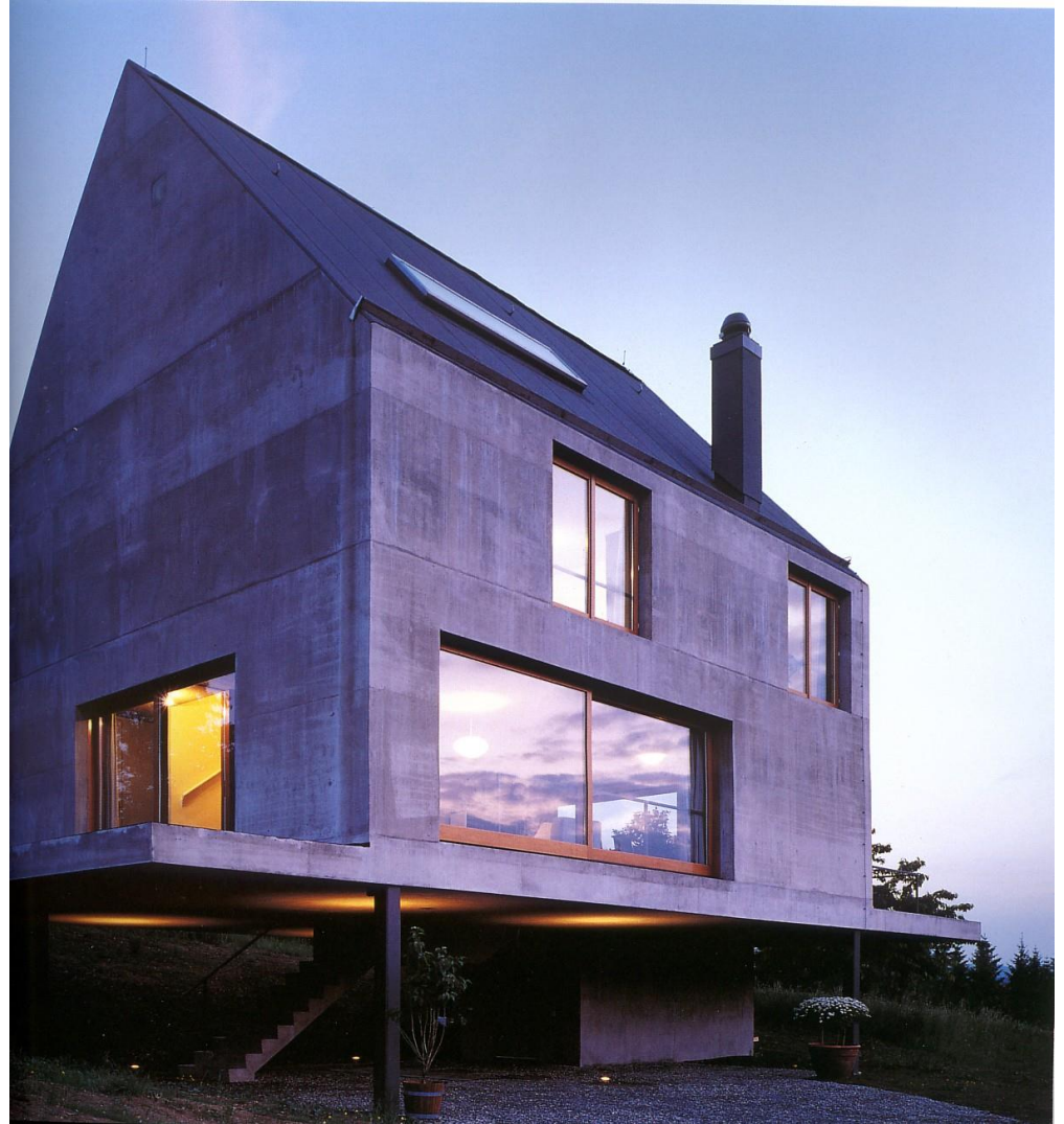
Rudin House, Leymen, France
