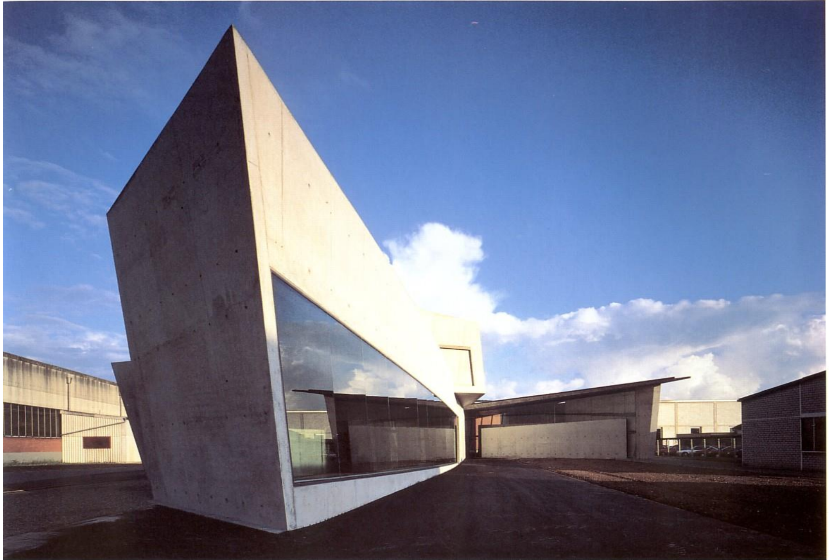
Vitra fire station
