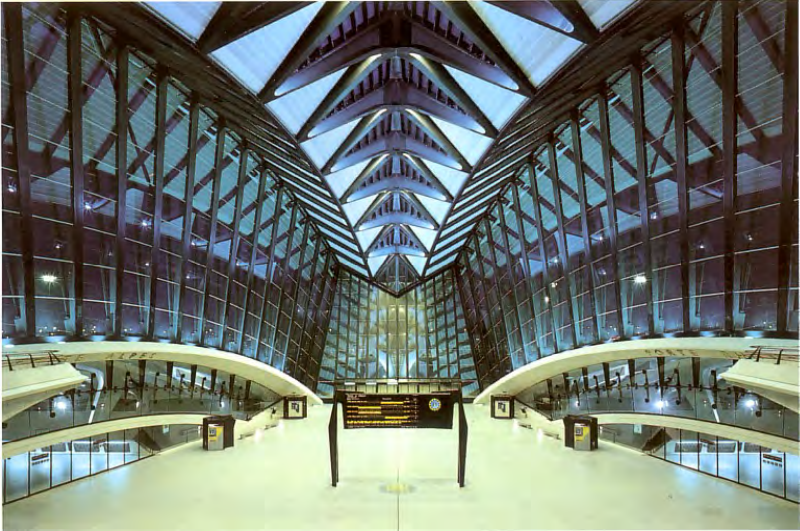
TGV Station, Lyon, France
