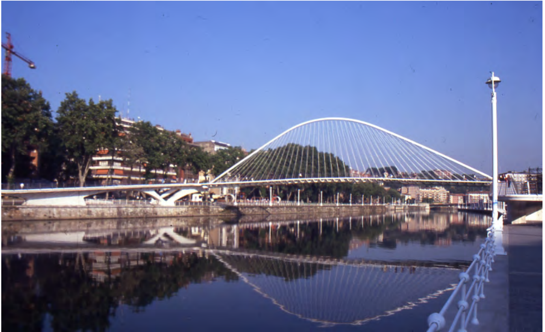
Bilbao Footbridge, Bilbao, France
