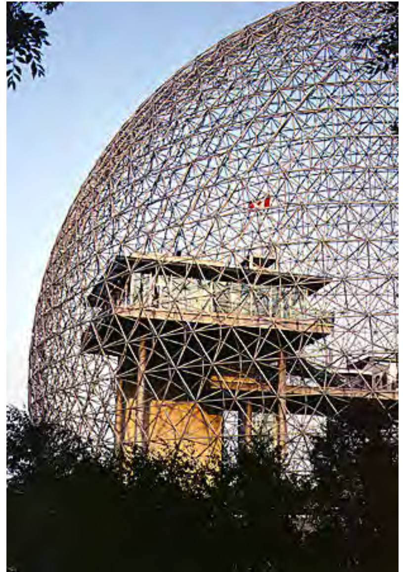
Geodesic dome, Montreal Fair, Montreal
