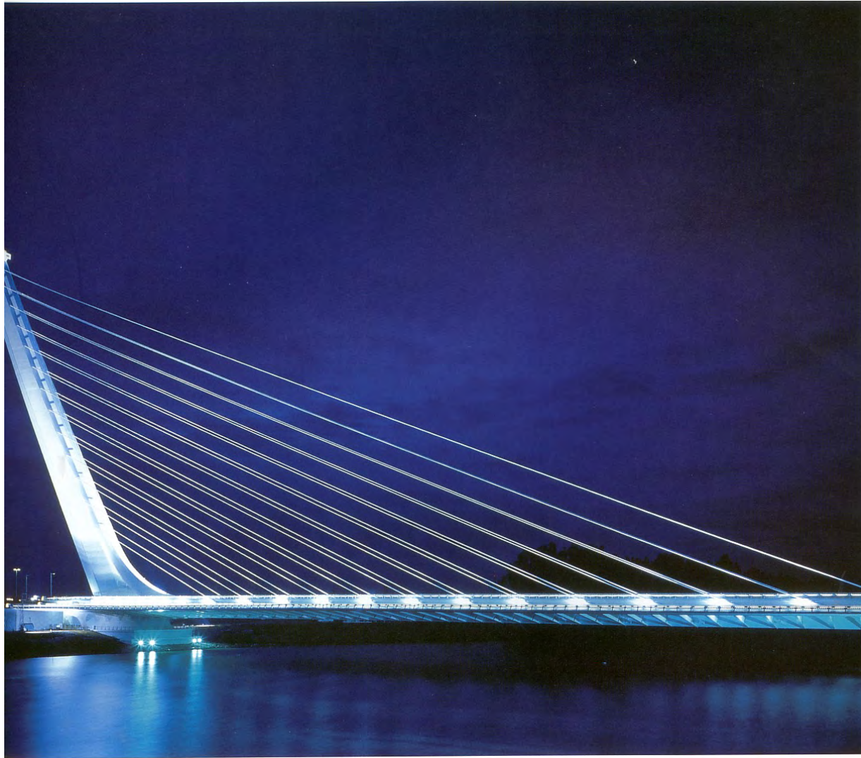
Alamillo Bridge, Seville
