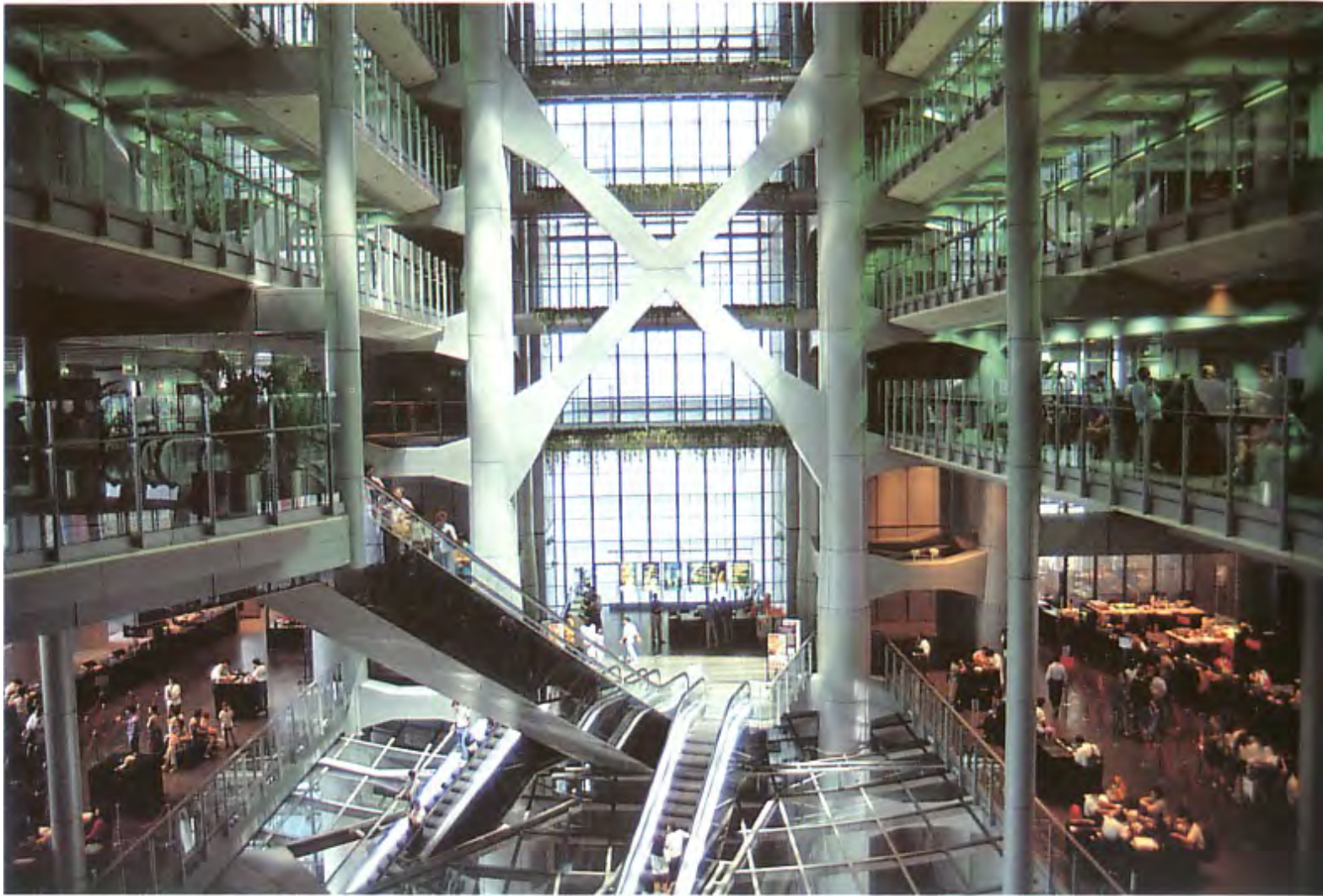
Hong Kong and Shanghai Bank, Hong Kong 1979-86
