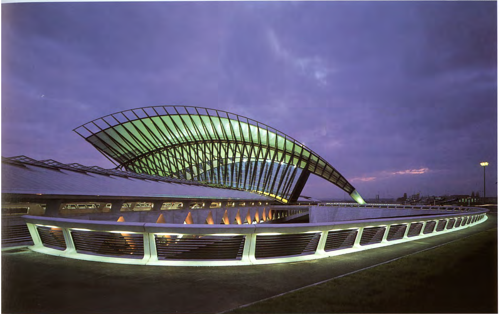
TGV Station, Lyon, France
