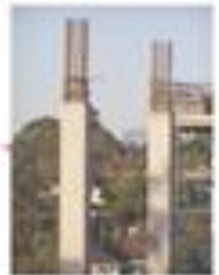
Thin exterior structural columns
