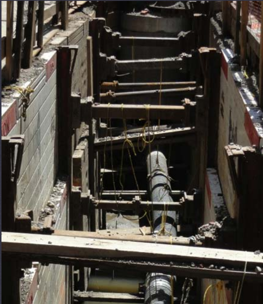
SOLDIER BEAMS & LAGGING
