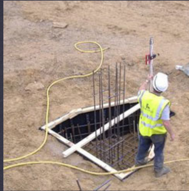
Pile Cap Casting
