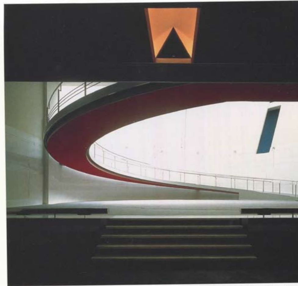
Spiral ramp leading to the second-floor shops. The thin profile of the ramp is achieved with a structure of built-up steel plates, and the ramp itself is supported by walls at only three points. The continuous stainless steel handrail was welded and polished on site to achieve a seamless finish.
