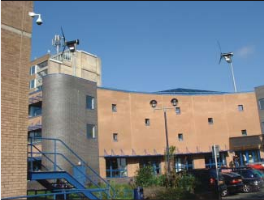
Two rooftop mounted Proven turbines
