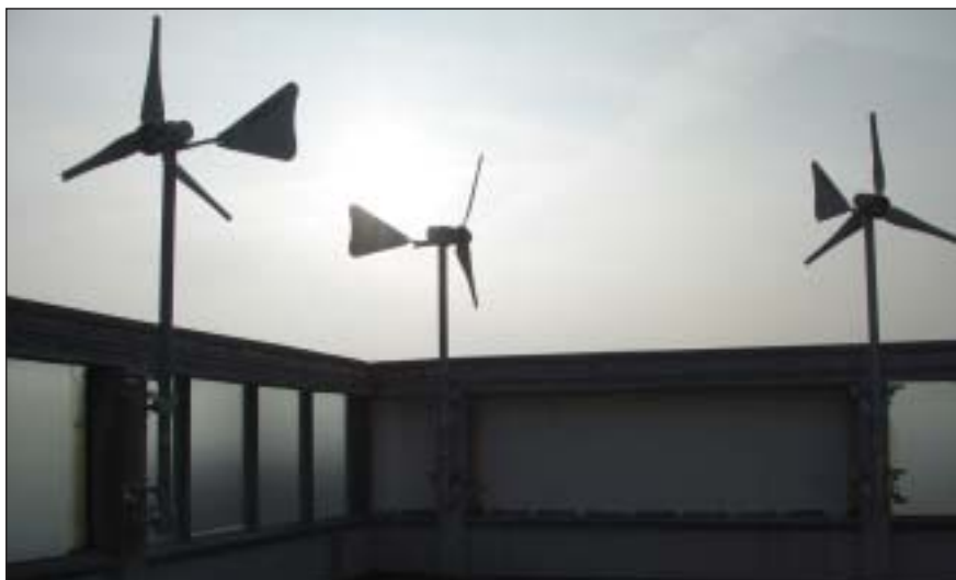
The recent installation at the CFS tower in Manchester
