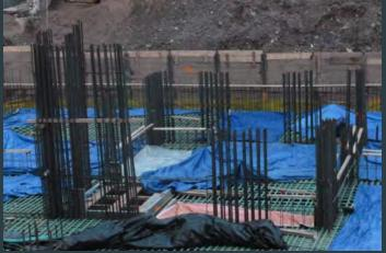
This looks like coated/treated rebar that will soon be set into poured concrete. The vertical rebar is untreated and will probably end up being columns or walls that will support the structure
