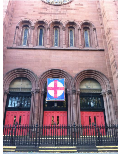
Left side entrance showing arch windows, and tall doors.
