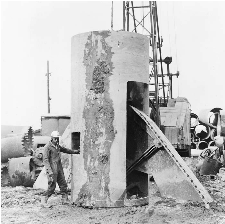
FIGURE 2.40 The bell is formed at the bottom of the caisson shaft by a belling bucket with retractable cutters. The example shown here is for an 8-foot- (2.44-m)-diameter shaft and makes a bell 21 feet (6.40 m) in diameter. (Courtesy of Calweld Inc.)
