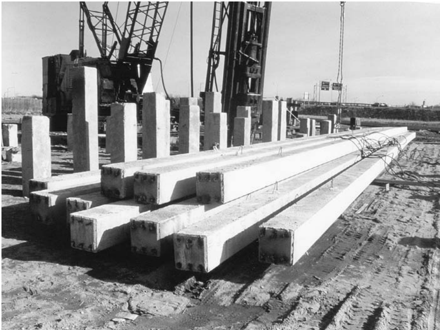
FIGURE 2.48 Precast, prestressed concrete piles. Lifting loops are cast into the sides of the piles as crane attachments for hoisting them into a vertical position. (Courtesy of Lone Star/San-Vel Concrete)
