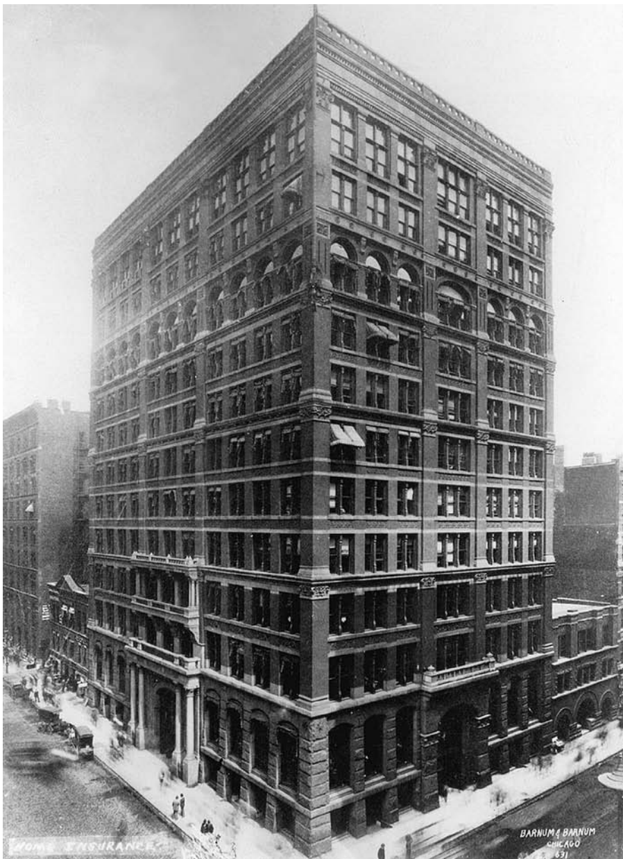
FIGURE 11.4 The Home Insurance Company Building, designed by William LeBaron Jenney and built in Chicago in 1893, was among the earliest true skyscrapers. The steel framing was fireproofed with masonry, and the exterior masonry facings were supported on the steel frame. (Photo by Wm. T. Barnum. Courtesy of Chicago Historical Society ICHi-18293)
