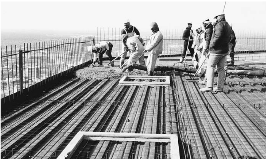
FIGURE 11.63 Composite beam construction.
