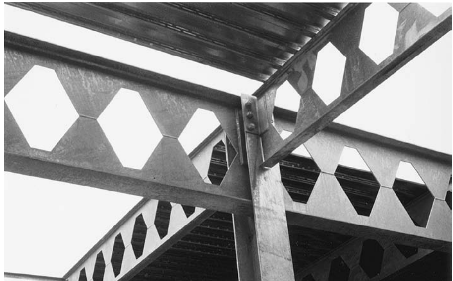
FIGURE 11.78 Castellated beams and girders frame into a wide-flange column. (Courtesy of Castelite Steel Products, Midlothian, Texas)
