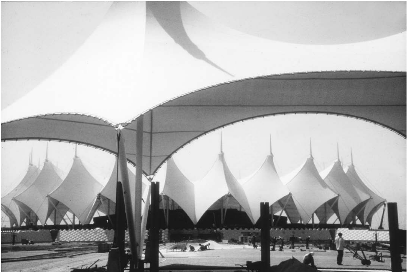
FIGURE G Like the petals of a giant flower, tensile structures arranged in a huge circle shade the grandstand of King Fahd Stadium in Riyadh, Saudi Arabia. The masts are 190 feet (58 m) high. (Architects: Ian Fraser, John Roberts & Partners. Roof designer and structural engineer: Geiger Berger Associates)
