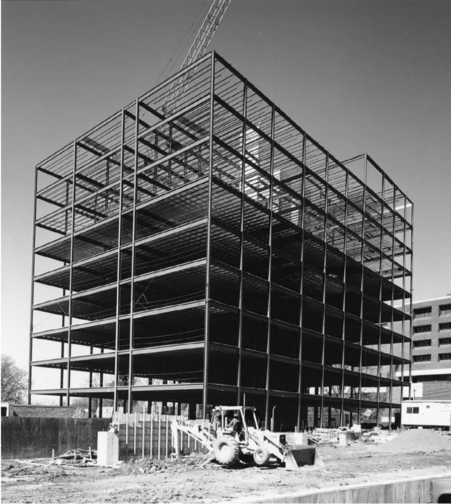
FIGURE 11.57 A 10-story steel frame nears completion. The lower floors have already been decked with corrugated steel decking. (Courtesy Vulcraft Division of Nucor)
