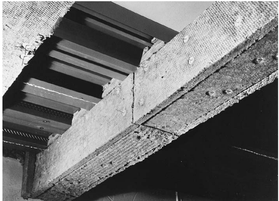
FIGURE 11.75 Slab fireproofing on a steel beam. (Courtesy of United States Gypsum Company)
