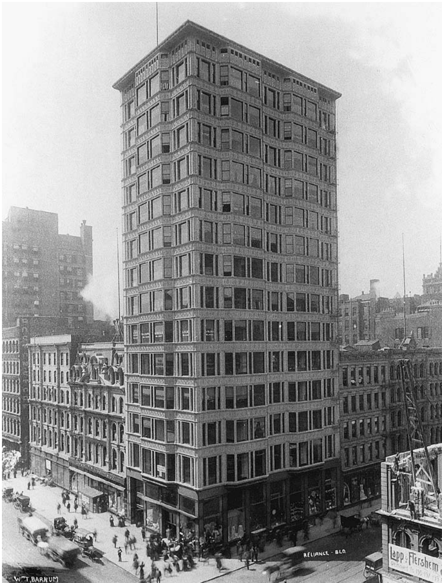
FIGURE 19.2 The curtain wall of Chicago's Reliance Building, built in 1894–1895, has spandrels constructed of white terra-cotta tiles. (Architect: Charles Atwood, of Daniel H. Burnham and Company. Photo by Wm. T. Barnum. Courtesy of Chicago Historical Society ICHi-18294)
