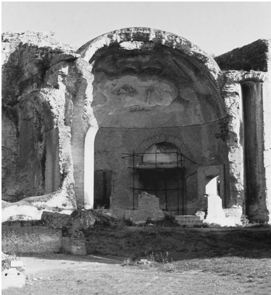
FIGURE 13.2 Hadrian's Villa, a large palace built near Rome between A.D. 125 and 135, used unreinforced concrete extensively for structures such as this dome. (Photo by Edward Allen)
