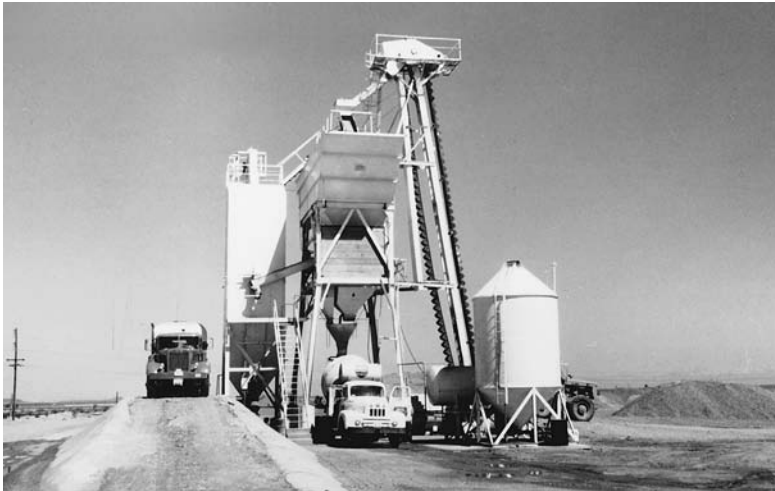
FIGURE 13.9 Charging a transit-mix truck with measured quantities of cement, aggregates, admixtures, and water at a central batch plant. (Reprinted with permission of the Portland Cement Association from Design and Control of Concrete Mixtures, 12th edition; Photos: Portland Cement Association, Skokie, IL)
