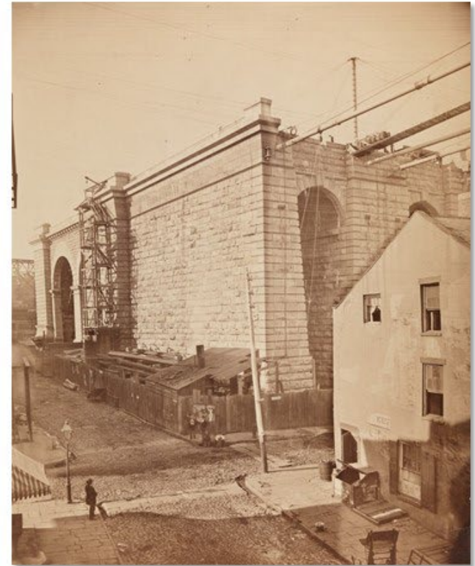
The Anchorage visible from the outside with masonry walls. The cables enter at top.
