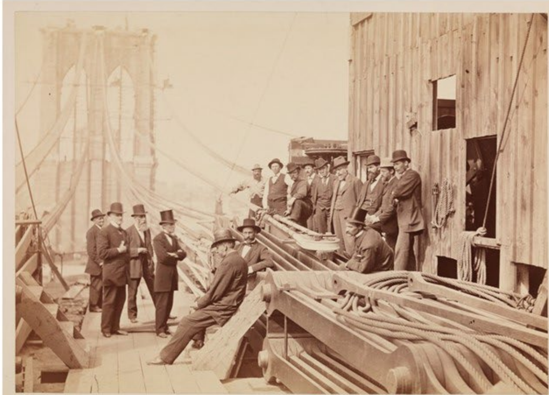
October 1878 - Brooklyn Anchorage - Shows the anchor chains as they extend and transition to the suspension cable strands. Note one of the strands looped around a cast iron shoe rotated horizontally during the spinning & the travelling wheel.
