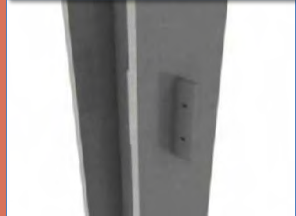
Beam to Column Fin Plate
