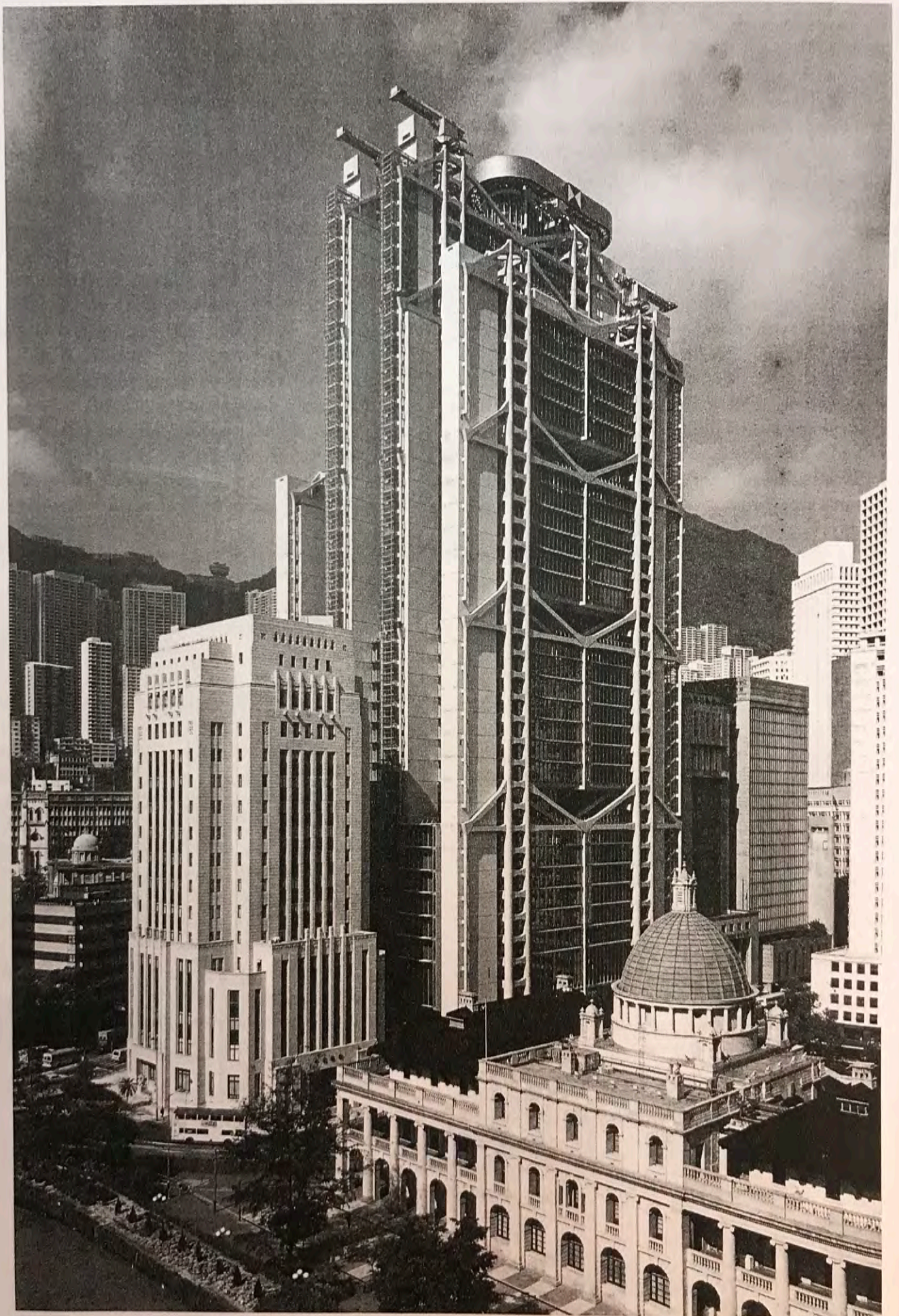
20.28. Norman Foster, Hong Kong Shanghai Bank, Hong Kong, 1979–1985. In such megastructures the expressive force of engineering reaches its height. Photo: Ian Lambot/arcaid.co.uk.
