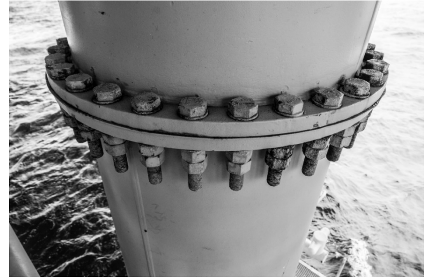
Bolted Structural connection
