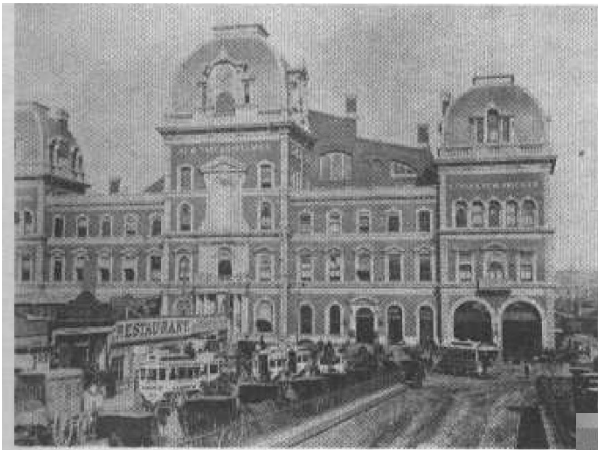
Park Avenue and Grand Central Depot from 41st Street, before 1886.
