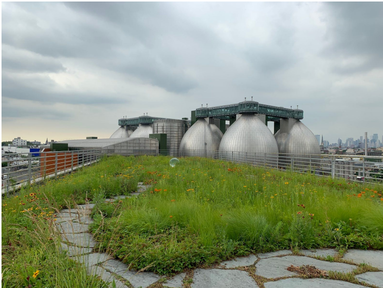
Green Roof surrounded by the industry
