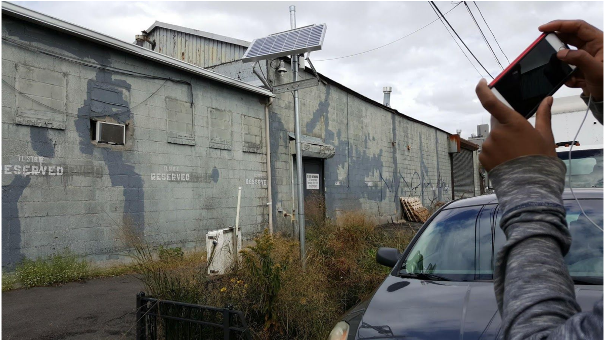
Solar Panels; These solar panels were found also right in the middle of the rain gardens. It's also located on 2nd Avenue between 5th and 6th street. Solar panels absorb sunlight as a source of energy and then utilizes it to generate electricity.
