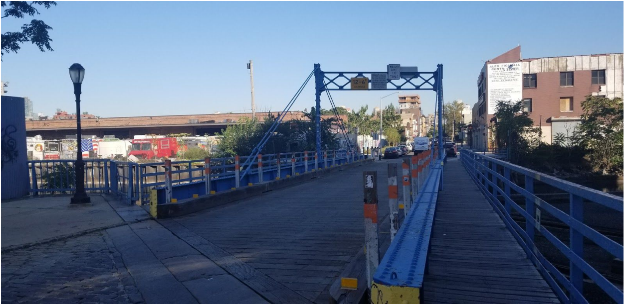
Carroll Street Bridge in its stable position, when not used as a moveable bridge.
