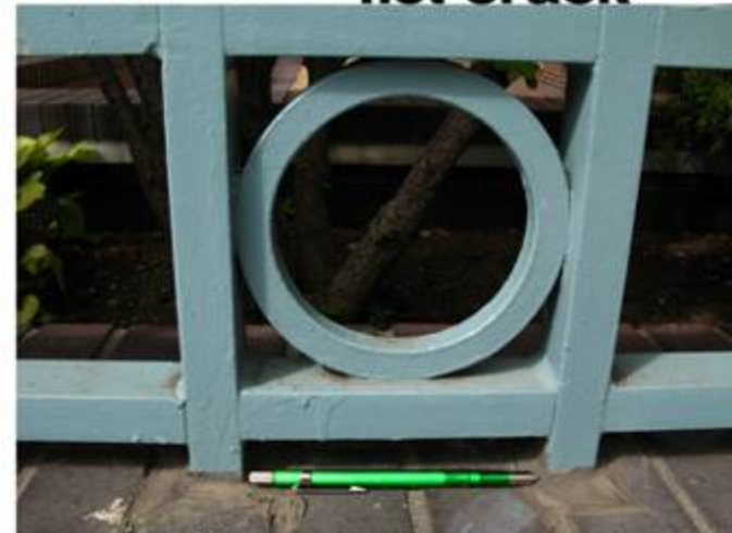
allows for expansion & contraction so joint will not crack
