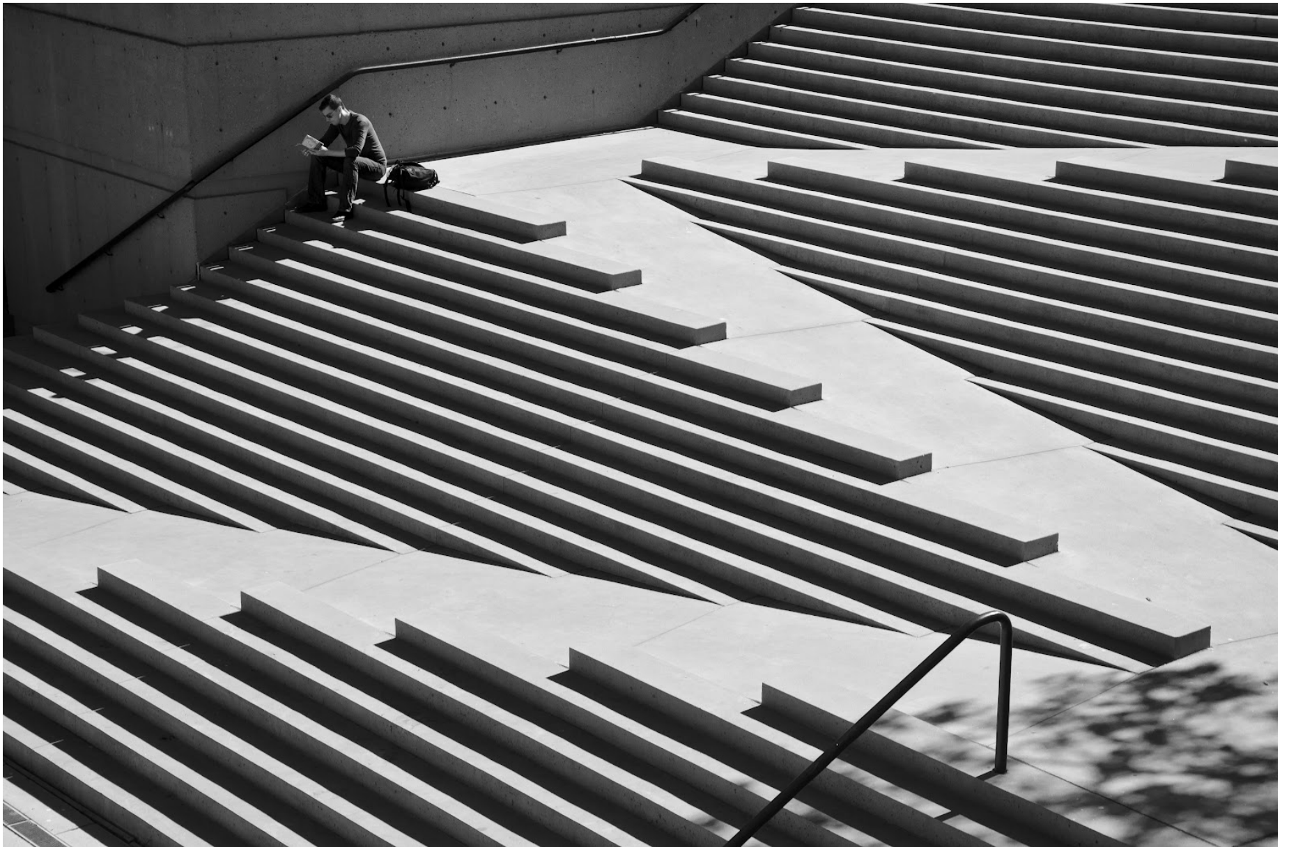
Robson Square in Vancouver for wheelchair accessibility
