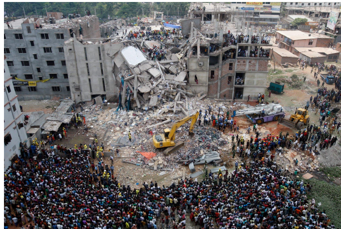
Figure 2: A photo from 2013 shows rescue workers at the site of the eight-story building Rana Plaza which collapsed at Savar, outside Dhaka, Bangladesh.
