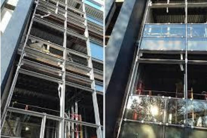
Stick curtain wall are processed, manufactured at factory and assembled, installed and completed at site. This kind of curtain wall can be used for all outside surface system types of buildings.
