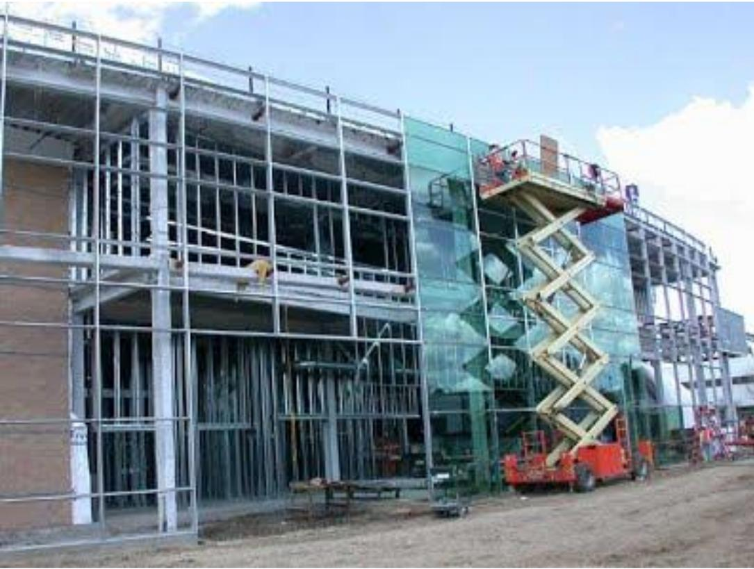
The self weight of the curtain wall is normally taken to the round thorough the mullions. Mullions spacing are normally in the range of 1.2 to 2 meters Wider spacings are possible. Transom spacings are normally determined by panel requirements
