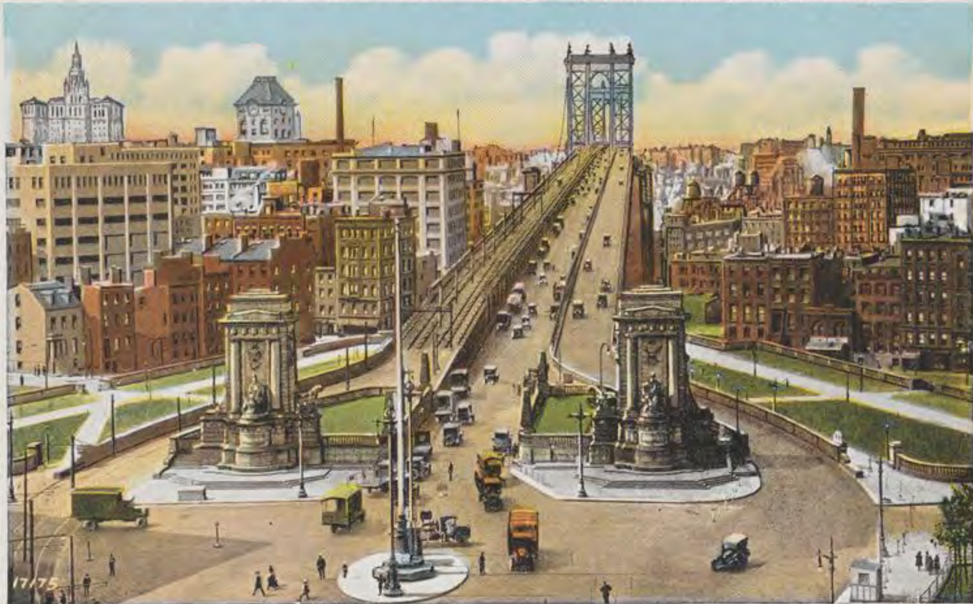
Bird's-Eye View of the Manhattan Bridge Approach, Brooklyn, N. Y.
