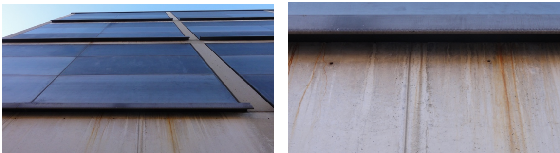
Figure 12. Inquiry and Research: Student photographs of observations of condensation stains emitted from behind exterior metal panels and drip profile, Yale Center for British Art, 2014.
