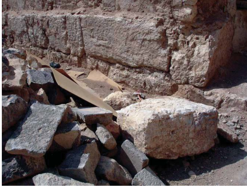
Figure 13 Detail of the southern side of the ashlars in the southernmost bedroom (possible iwān ) of the service courtyard in 2006, view looking northwards. Note the continuation of the lower course of ashlars to the east (S. Weber).
