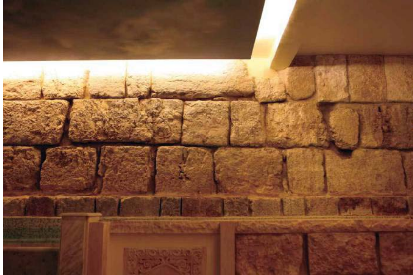
Figure 9 Easternmost section of the basement wall (G. H. Lewis).
