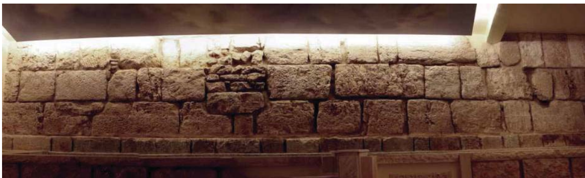
Figure 6 Wall in the basement of Bayt Farhi with the edge of the lap pool in the foreground (G. H. Lewis).
