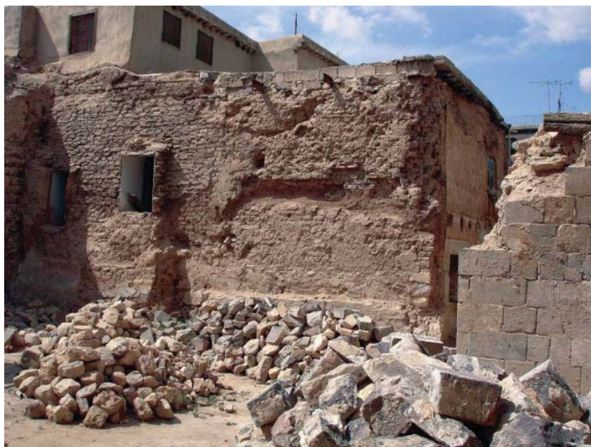
Figure 12 The south face of the ashlar in the southernmost bedroom (possible iwān ) of the service courtyard in 2006, view looking northwards (S. Weber).
