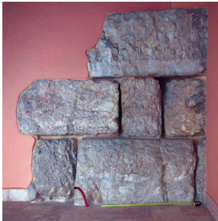
Figure 16 Detail, southern section of the wall in Fig. 13, south-eastern bedroom, the service courtyard (G. H. Lewis).
