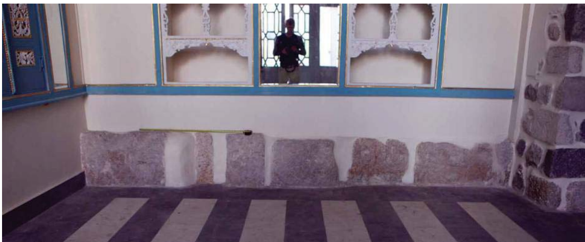
Figure 10 Eastern section of the wall in the southernmost bedroom (possible iwān ) of the service courtyard (G. H. Lewis).
