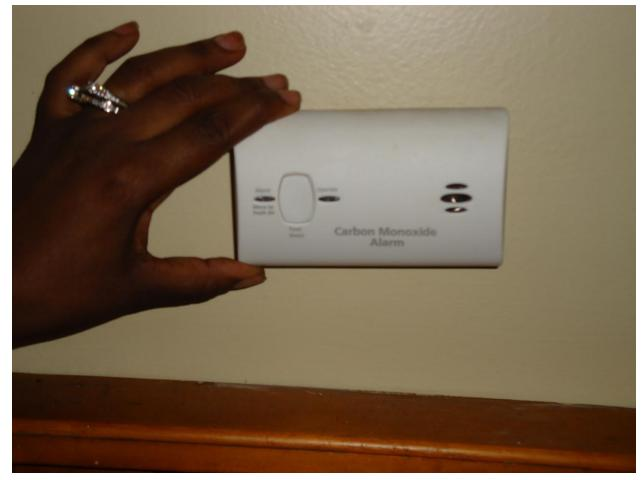
STEP9. PLEASE PRESS THE BUTTON ON THE CARBON MONOXIDE ALARM/DETECTOR TO MAKE SURE THAT IT IS INSTALLED PROPERLY. ENSURE THAT YOU HEAR THREE BEEPS TO KNOW THAT YOU HAVE SUCCESSFULLY INSTALLED THE CARBON MONOXIDE ALARM/DETECTOR. GIVE YOURSELF A TAP ON THE BACK FOR A JOB WELL DONE!!!!!! NOW BE SAFE CAUSE REMEMBER SAFETY FIRST.
