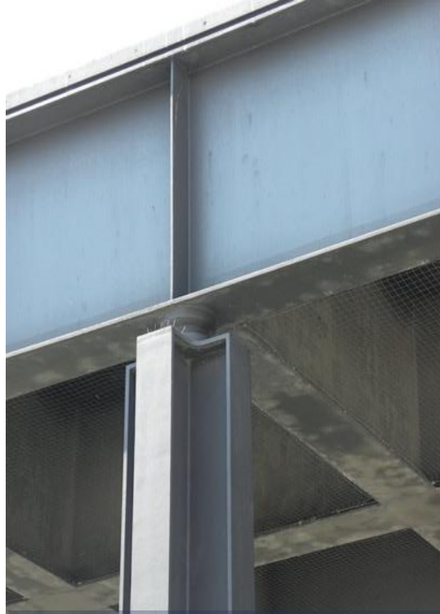
16. Details of column and pin-joint.
