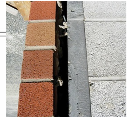
Wall Section: Reinforced Concrete Block Cavity Wall
