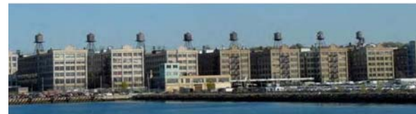
Adapting green building concepts to Sunset Park (Artist impression by DSA and JA Architecture)
