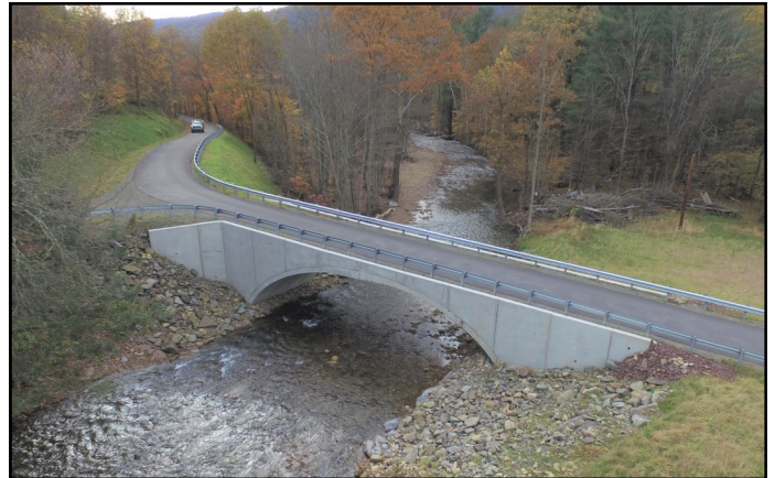
Upper Bodines Road Bridge, Lewis Township
