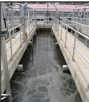
WW Treatment Plant Replacement, Millville Borough
