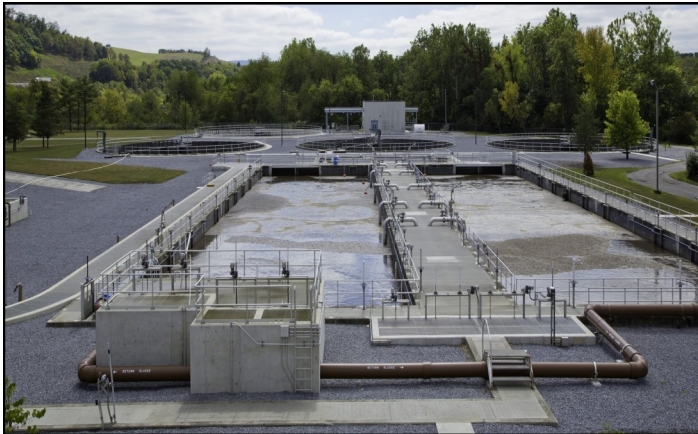
Altoona Water Authority, Westerly WWTF
