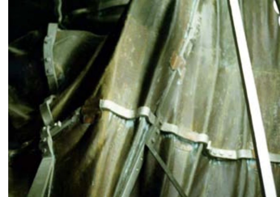
The Statue of Liberty is made from 300 sheets of hammered copper, held together by rivets. Each sheet is 3/32" thick, about the thickness of two pennies. During the restoration, seams between the sheets were carefully cleaned, then closed with a silicone sealant.
