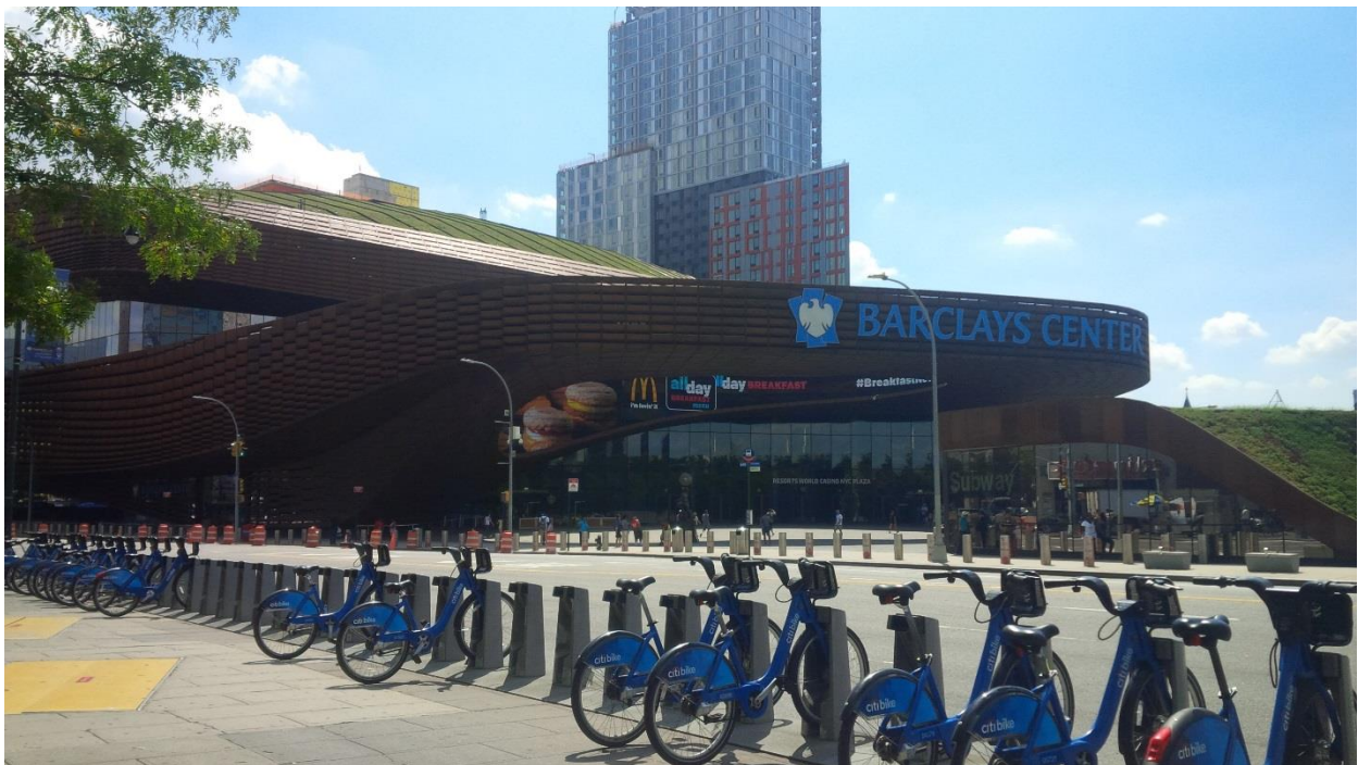
Image showing the entrance, types of materials used, and the green roof.
