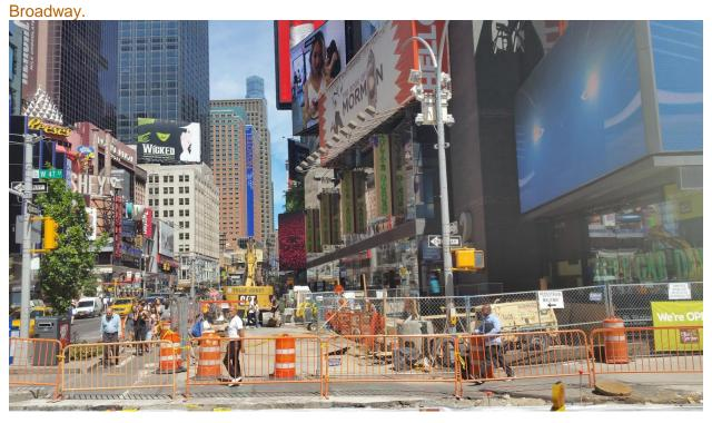
These two guys are taking a break from brick laying. They told me that they were replacing the sidewalk with bigger brick which would increase the width for more sitting area.
