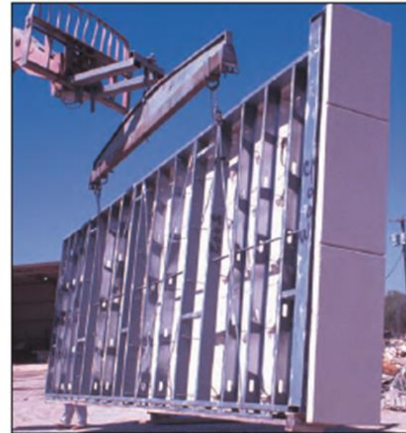
The GFRP skin includes a corner return that provides a means of forming sealed joints between panels. A minimum 2-in. return is required. A larger return may be needed for a two-stage joint between panels.
