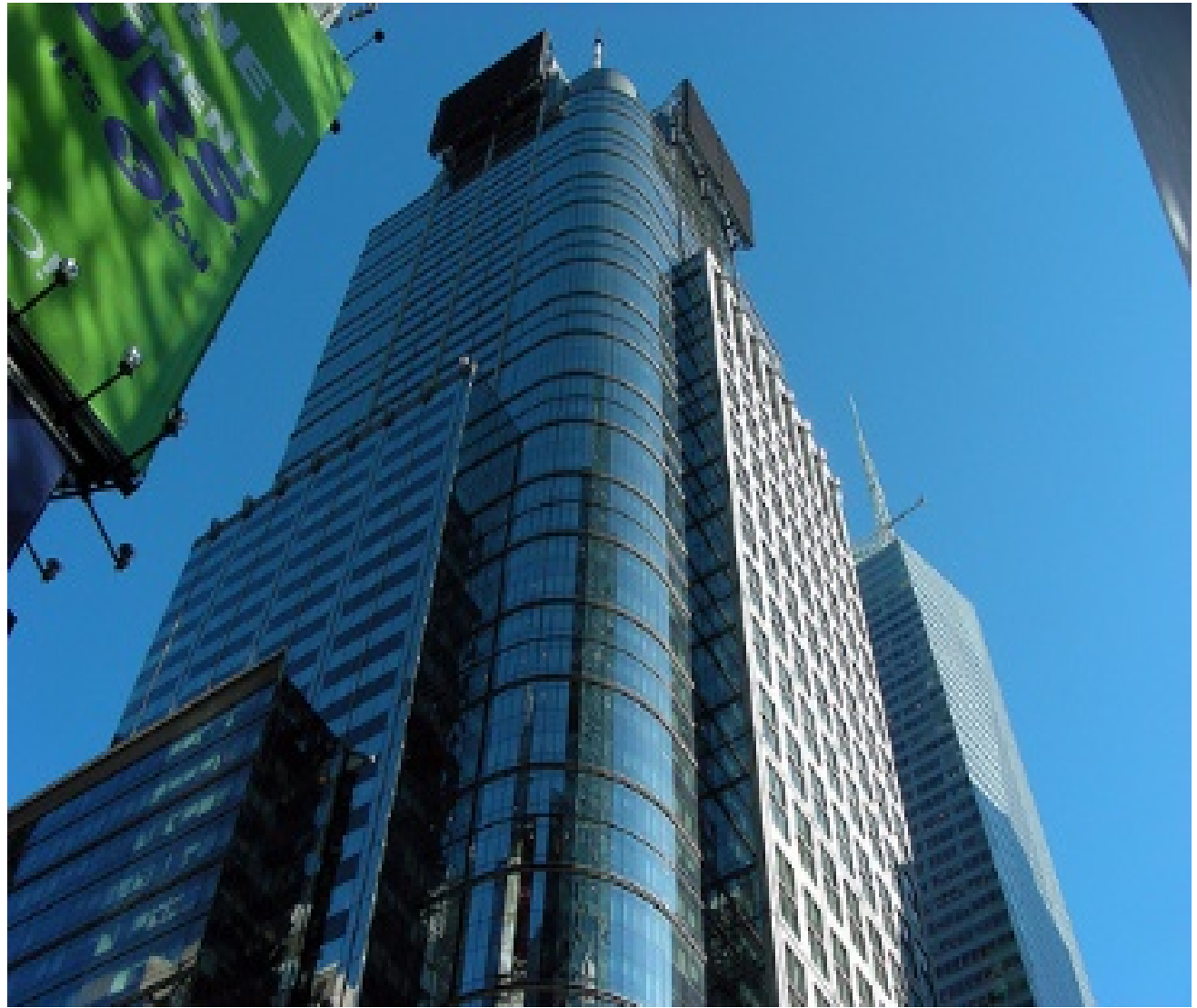
4 Times Square NY Office Building
