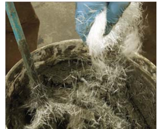
Adding fibres to concrete mix
