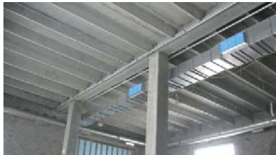
Structural Component: Double Tee
