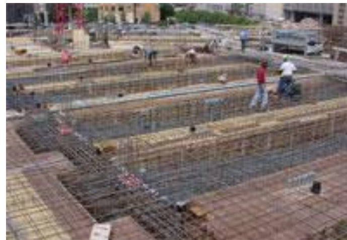
Post-tension transfer beams and tendon profiles..
