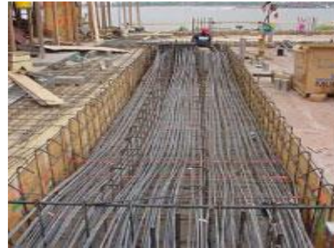
Monostrand tendons in a post-tensioned beam being laid out.
