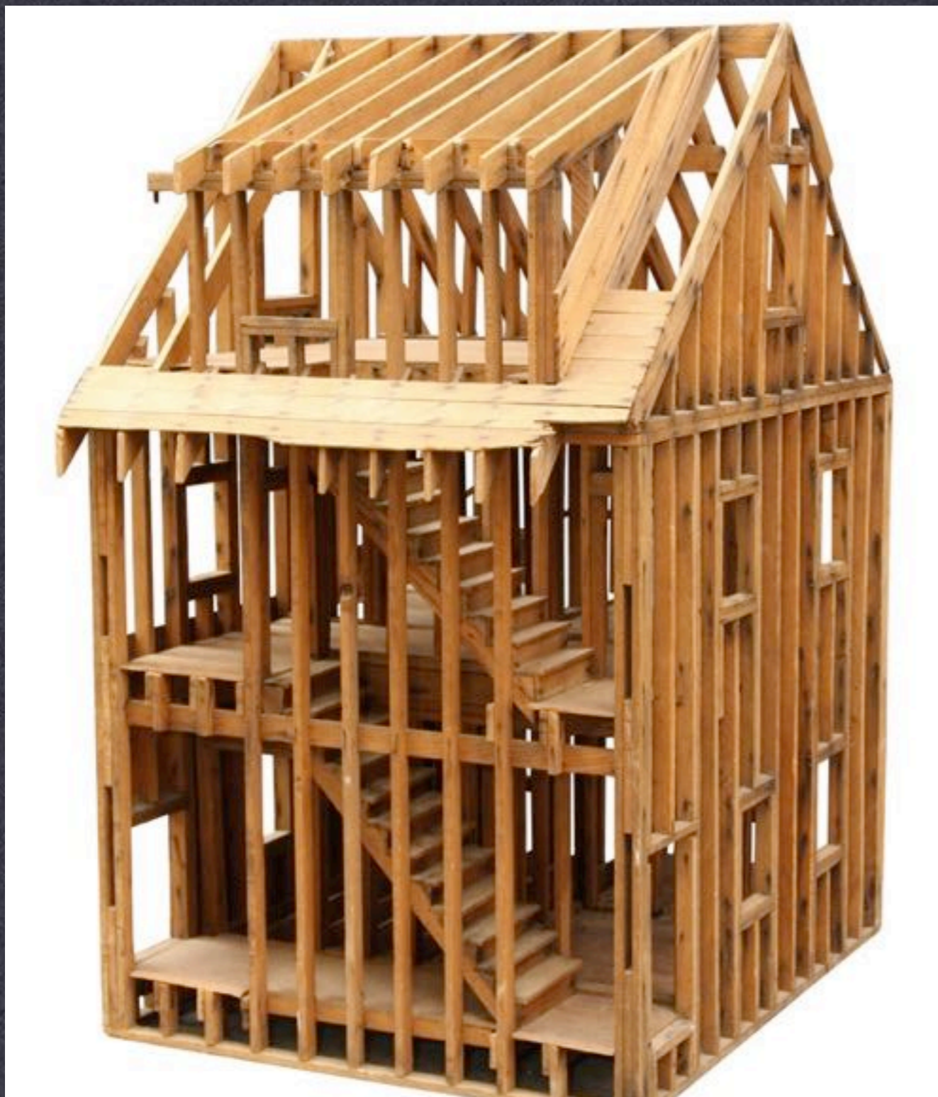
BALLOON FRAME CONSTRUCTION
