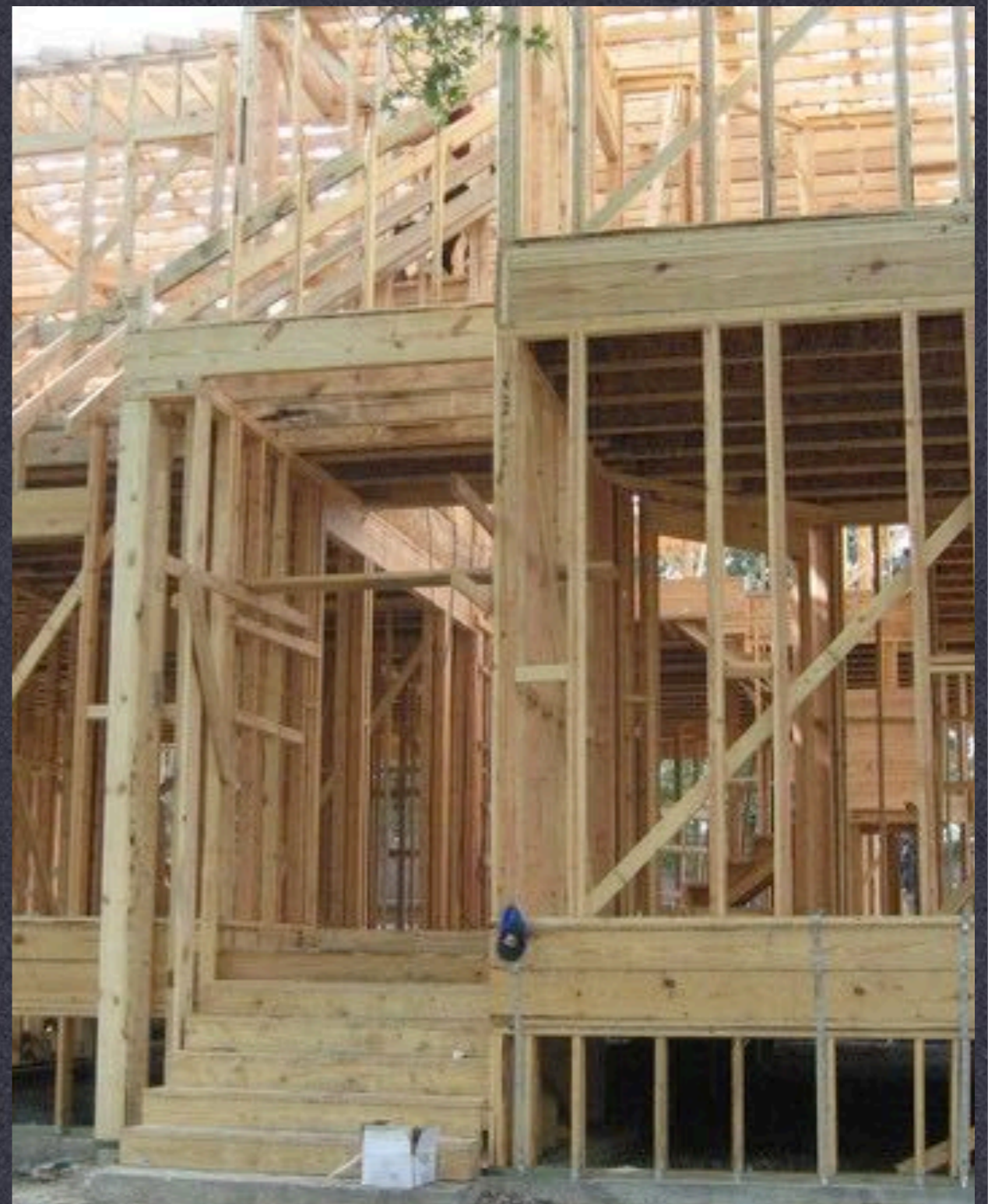
PLATFORM FRAME CONSTRUCTION
