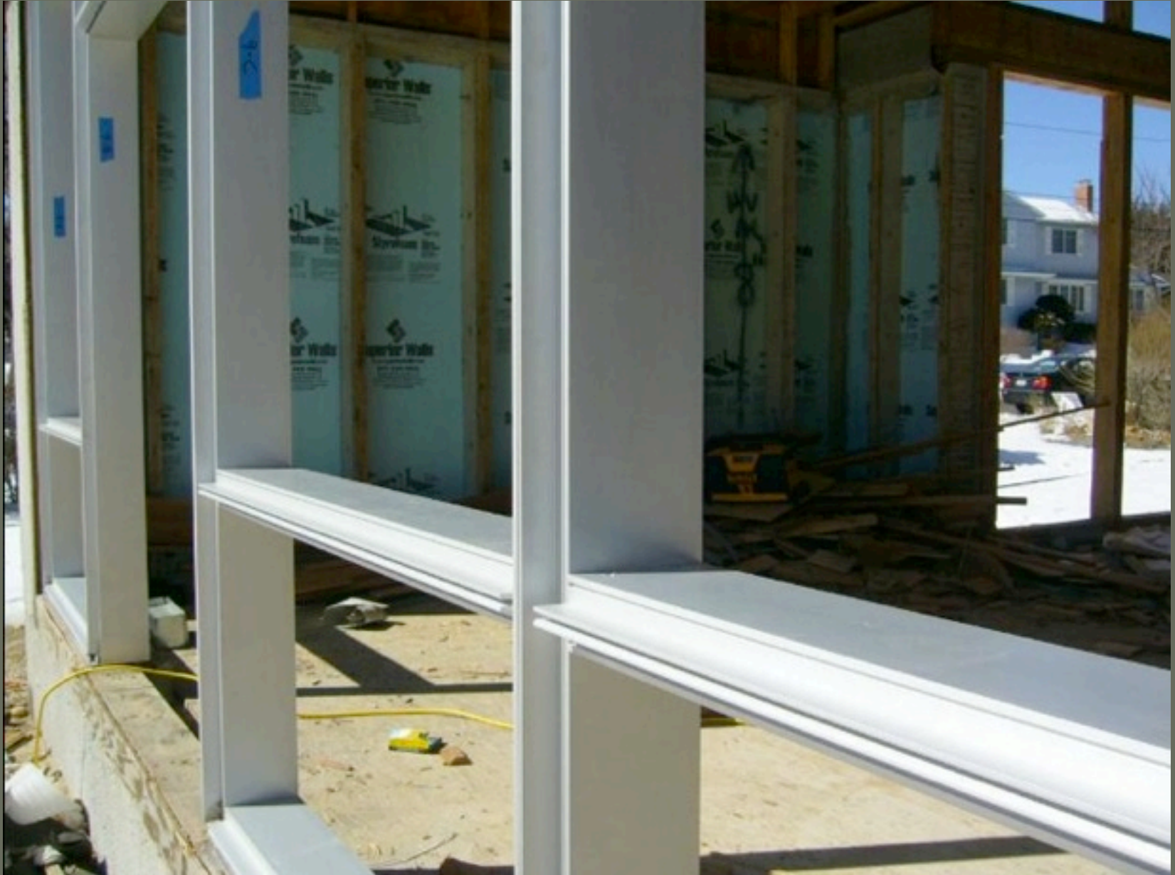
Curtain Wall Systems: stick system framing
